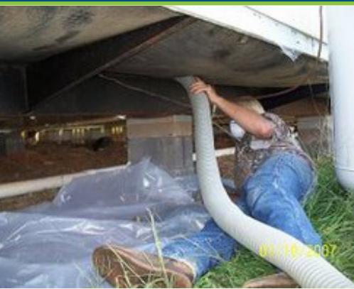
Weatherization technician installs insulation to the underbelly of a mobile home.
