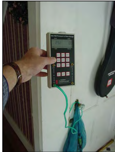
Zone pressure test to basement with blower door depressurizing house to -50 Pascals
